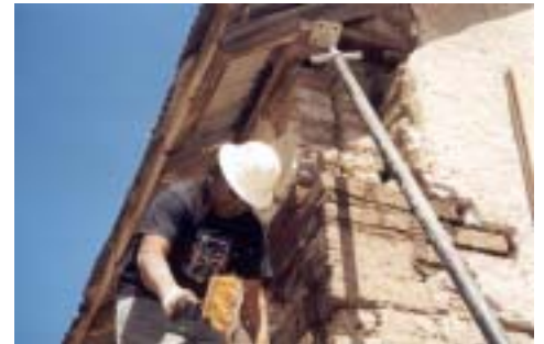
Means Design specialist makes adobe repairs to adobe haybarn SE corner.
