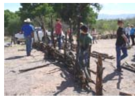
Retaque fence under construction (photos: C. Auerbach)
