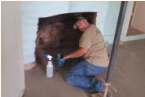
Marty Bond and Elyane Rocheford help clean the Ranch House; John Bellingham and Lucinda Iverson patch adobe walls and chimney. [photos: C. Auerbach]
