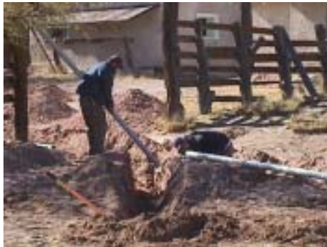
BLM fire crew member Jason McClain lays conduit in trench dug through main corral.
