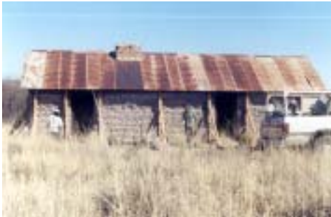
Completed shorings. (photos: L. Schupp)
