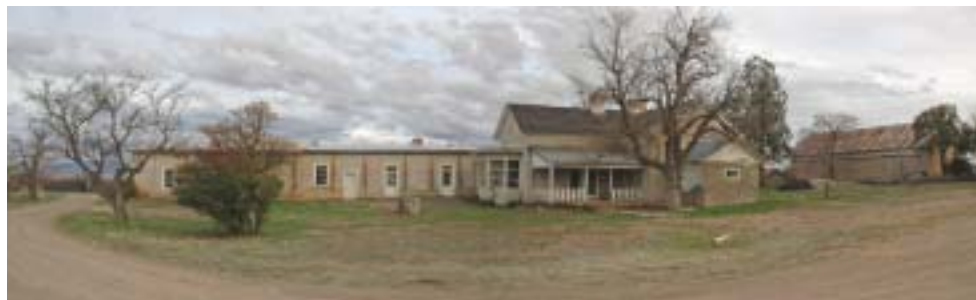
Empire Ranch House and Adobe Haybarn viewed from the West (photo: courtesy TuleReed.com Photography)
