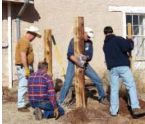
Volunteers set posts (photo: C. Martin)
