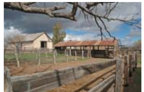
Repairing historic corrals will be a 2008 priority. (photo: CactusHuggers.com)
