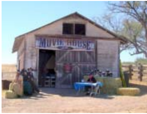
Newly repaired Mechanic's Shop donned a "Movie House" marquee for the Roundup, for screenings of John Wayne classic "The Cowboys."
