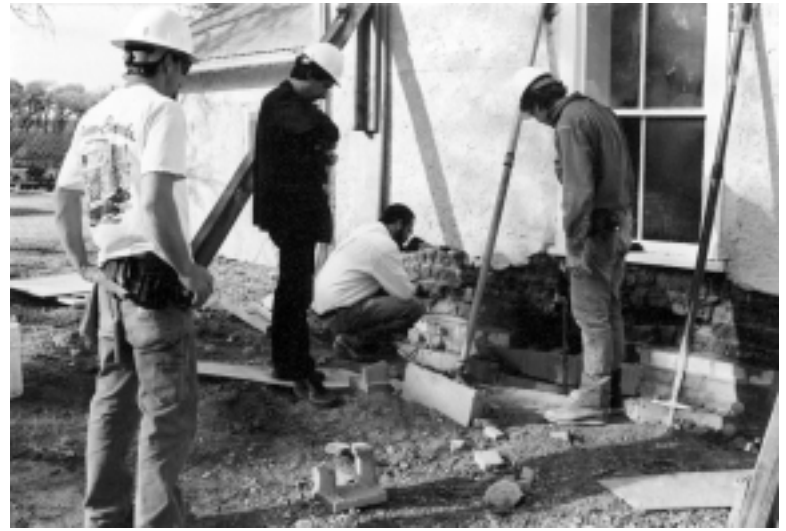
Foreman J. Barnett, architect B. Vint, ERF's S. Leidner, and E. Means inspect underpinning of bedroom foundation. (Photos: SRI)
