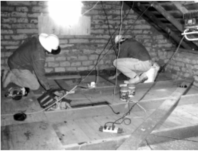
K. Hapton and M. Carbone of Means Design at work bracing and anchoring the roof above Victorian Addition living room.
