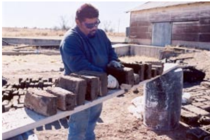
Francisco Montano of Means Design and Building Corp. hand casts replacement adobe for ranch house. (Photo: M. Witkind)
