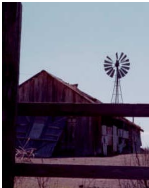
Horse barn and wind mill, north view from ranch house front yard (Photo: Laurel Wilkening, Mar. 2001)
