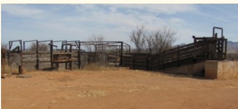
Volunteer stains replacement corral posts (left); the covered feed troughs (top); Adobe Haybarn east door (center); and Howe scale at shipping corrals (bottom) are next in line. (photos: BLM and S. Reichardt)
