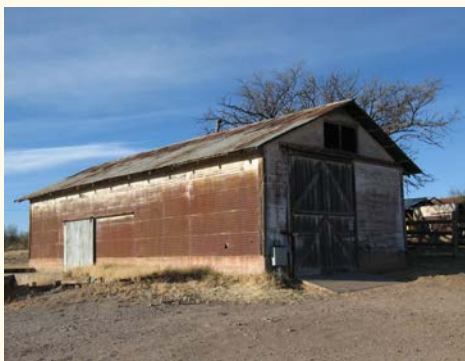
Mechanics Shed/Feed Barn exterior view (photo: K. Timmerman)
